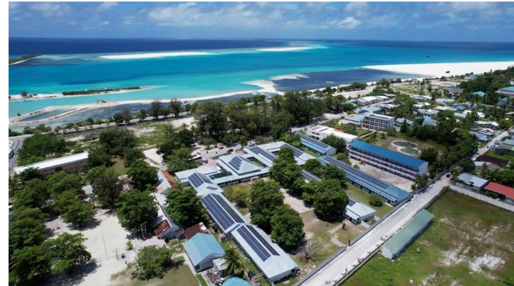
Renewable Energy Installation in Maldives
