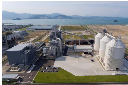
Biomass Power Plant
