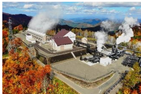
Geothermal Power Plant
