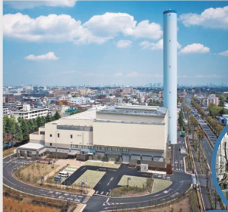
WtE plant (Clean Plaza Fujimi)
