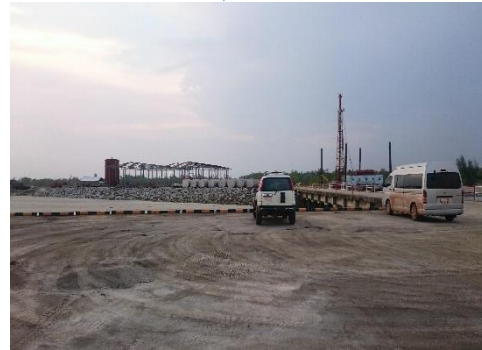
infrastructures in Myanmar
