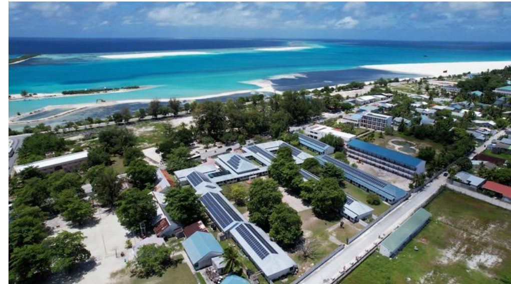
Renewable Energy Installation in Maldives
