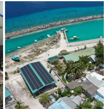
Solar PV at the project site
