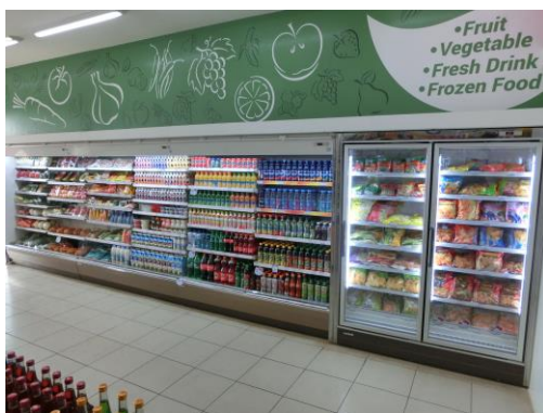
Energy saving at convenience stores, Panasonic, Indonesia
