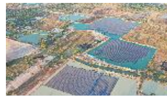
Floating Solar PV, TSB Co., Ltd., Thailand
