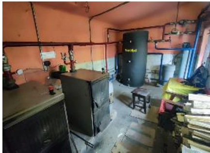
Wood boiler to A2W
