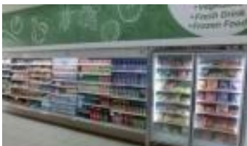
Energy saving at convenience stores, Panasonic, Indonesia
