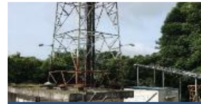
Energy-saving of mobile communications base transceiver stations, KDDI Corp. Indonesia
