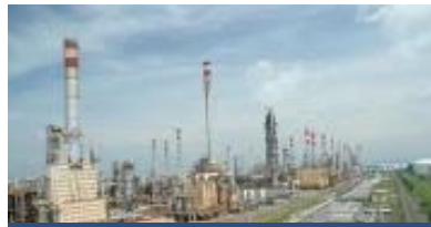
Optimization in petroleum refining plant, Yokogawa Electric Corp. Indonesia
