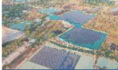
Floating Solar PV, TSB Co., Ltd., Thailand
