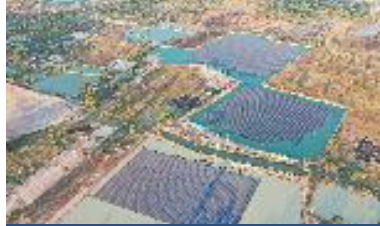
Floating Solar PV, TSB Co., Ltd., Thailand
