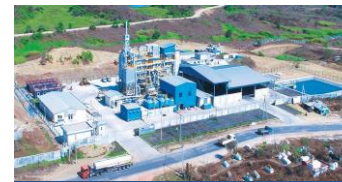
Waste to Energy Plant, JFE engineering, Myanmar
