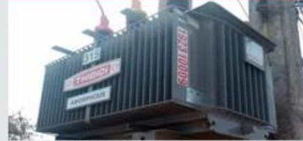
Amorphous Transformers (Lao PDR) Yuko Kelso Co., Ltd.
