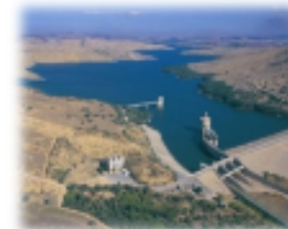
Support for dam upgrading project formulation (Tunisia)
