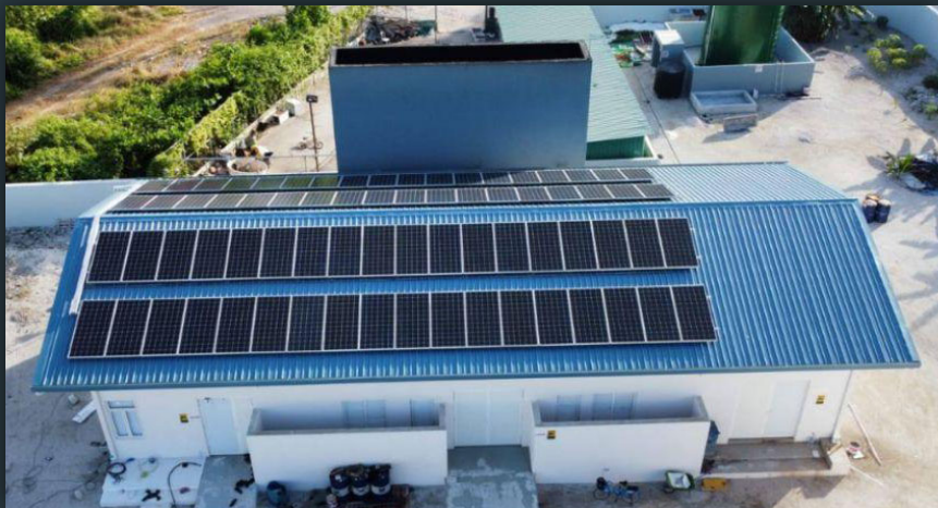
The 1 of many newly built Fenaka powerhouses to have solar installed on to power the entire building (26.28 kWp system on N.Miladhoo ) 3
