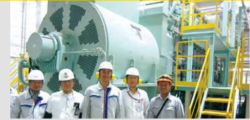
Gas Co-generation system (Indonesia)/ Toyota Tsusho Corporation
