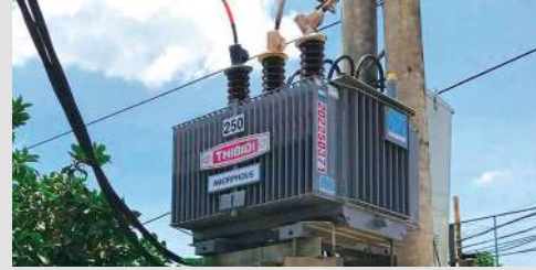
Amorphous Transformers (Viet Nam)/ Yuko Keiso Co., Ltd.
