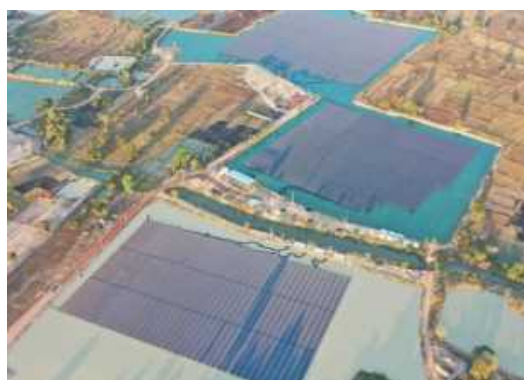
Floating solar power (Thailand) 2,552 tCO 2 /y. Start operation Jan. 2020
