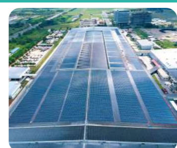
Philippines / Sharp Energy Solutions Corporation Solar PV
