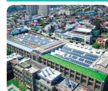
Chile / Waseda Environmental Institute Co., Ltd. Solar PV
