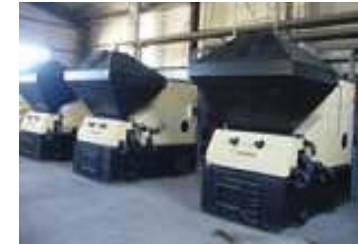
High-efficiency Heat only Boilers, Suuri-Keikaku, Mongolia
