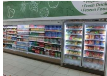
Energy saving at convenience stores, Panasonic, Indonesia
