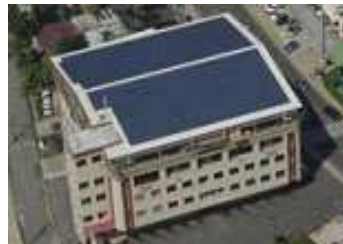
Installing solar PV system, PCKK, Palau Maldives
