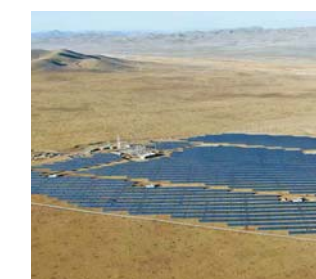
② Vicinity of New Airport 15MW + ADB Loan
