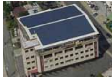
Installing solar PV system, PCKK, Palau Maldives
