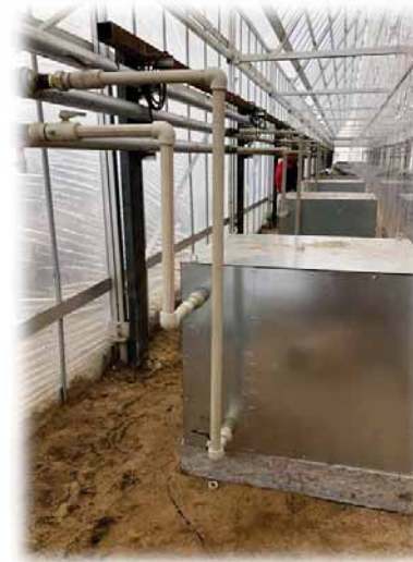
○ Air Handling Units
