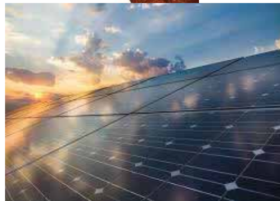
2. 10 MW Solar Energy
