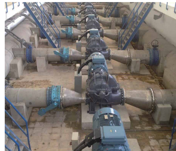
Replacement of high efficiency water pumps
