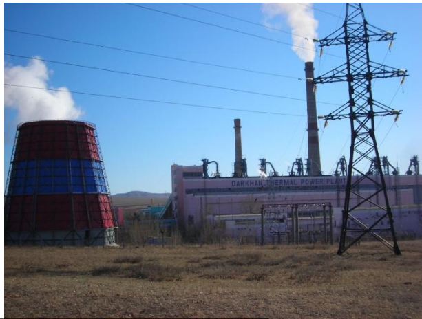
Darkhan CHP (48MW, 1965~)
