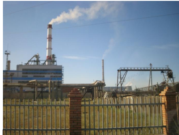
Thermal Power Plant #2 (24MW, 1961~)
