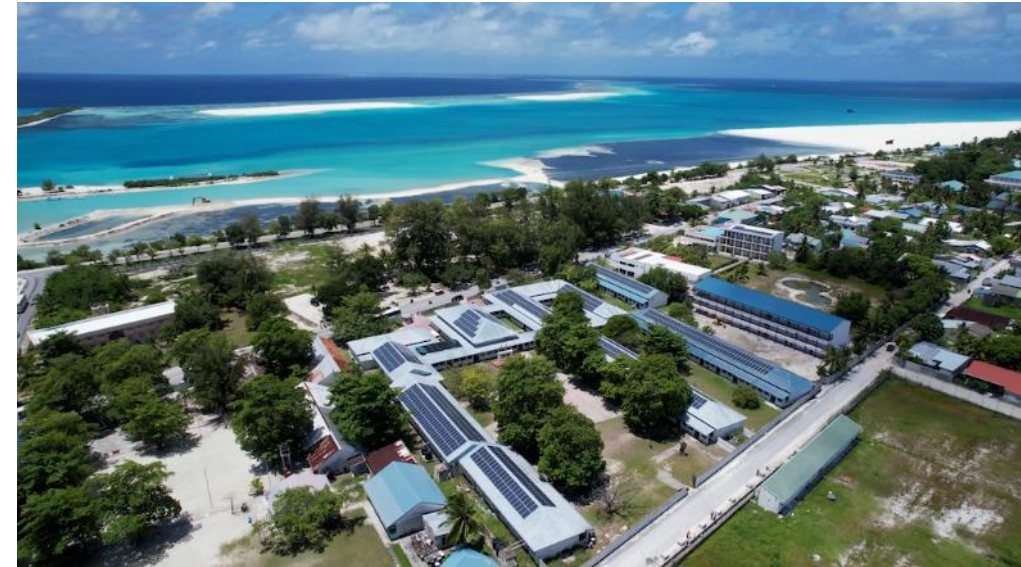
Renewable Energy Installation in Maldives
