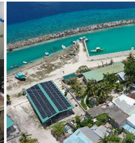
Solar PV at the project site
