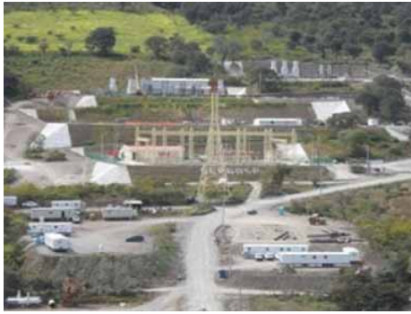
Geothermal power generation, Mitsubishi Hitachi Power Systems, Mexico
