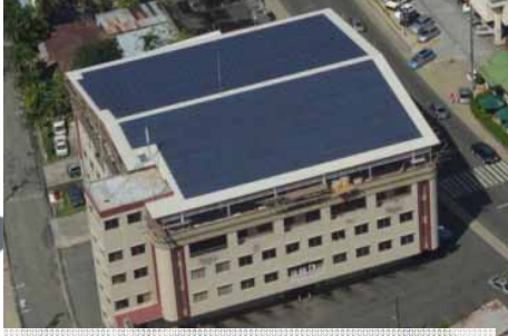
Solar power plant for commercial facilities, Kyocera, Palau
