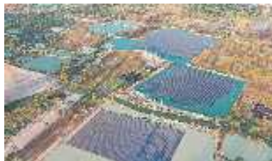
Floating Solar PV, TSB Co., Ltd., Thailand
