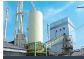
Biomass Co-Generation System, Fuji-Foods Coporation, Thailand
