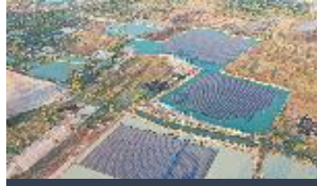
Floating Solar PV, TSB Co., Ltd., Thailand
