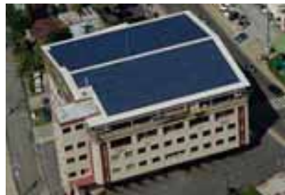
Installing solar PV system, PCKK, Palau Maldives
